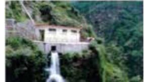
Small Scale Hydro Power Plant
