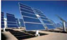
Solar Power Plant
